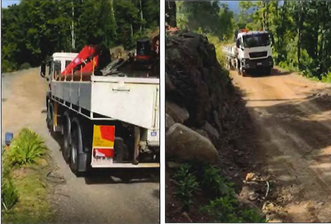
FIGURE 1.3 – GRADIENT AT THE BASE OF THE DRIVEWAY
