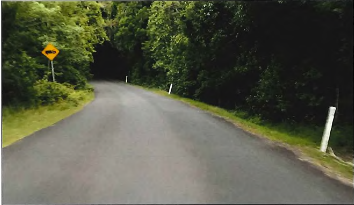
Existing Truck warning sign in southbound approach to curve
