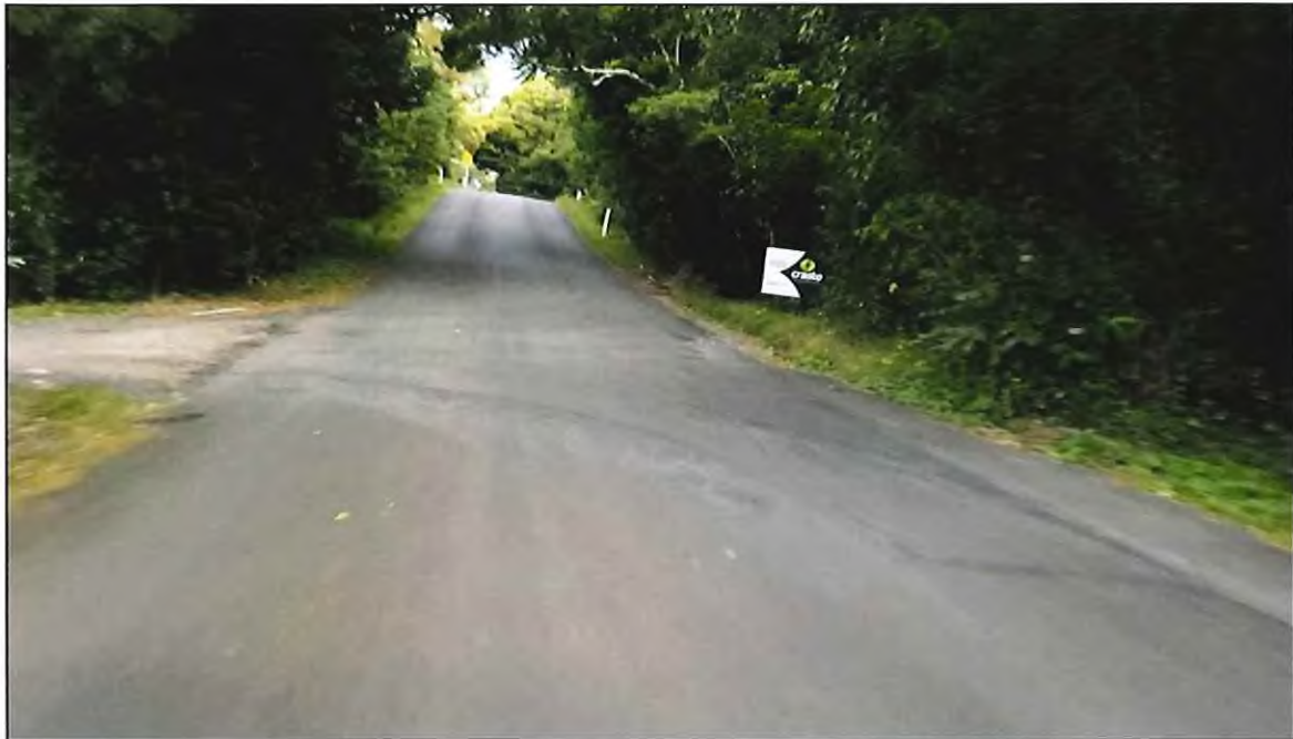
Sufficient width available for two vehicles to pass safely in low speed environment
