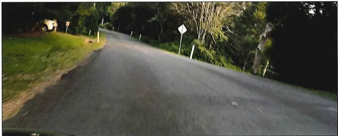
Section immediately south of Lyrebird Ridge Rd intersection
