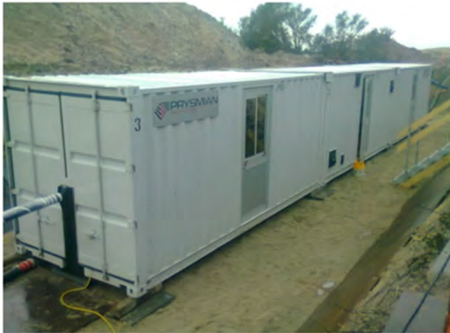
Figure 2-40. Photo of typical jointing containers (Source: Prysmian)
