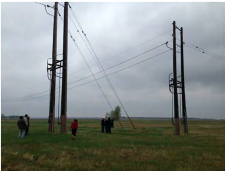
Figure 2-30. An Electrode Site Without a fence and electrode switches mounted on poles [CIGRE TB 675 Figure 7.4]
