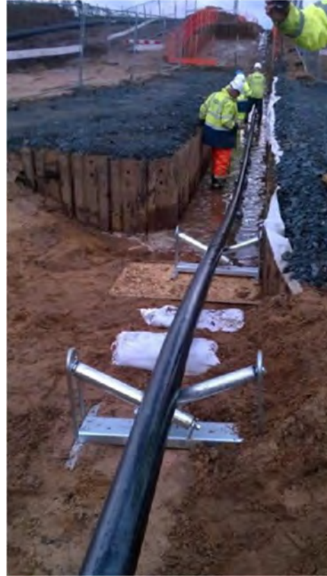
Figure 2-37. Photo of a sheeted trench (Source: Prysmian)
