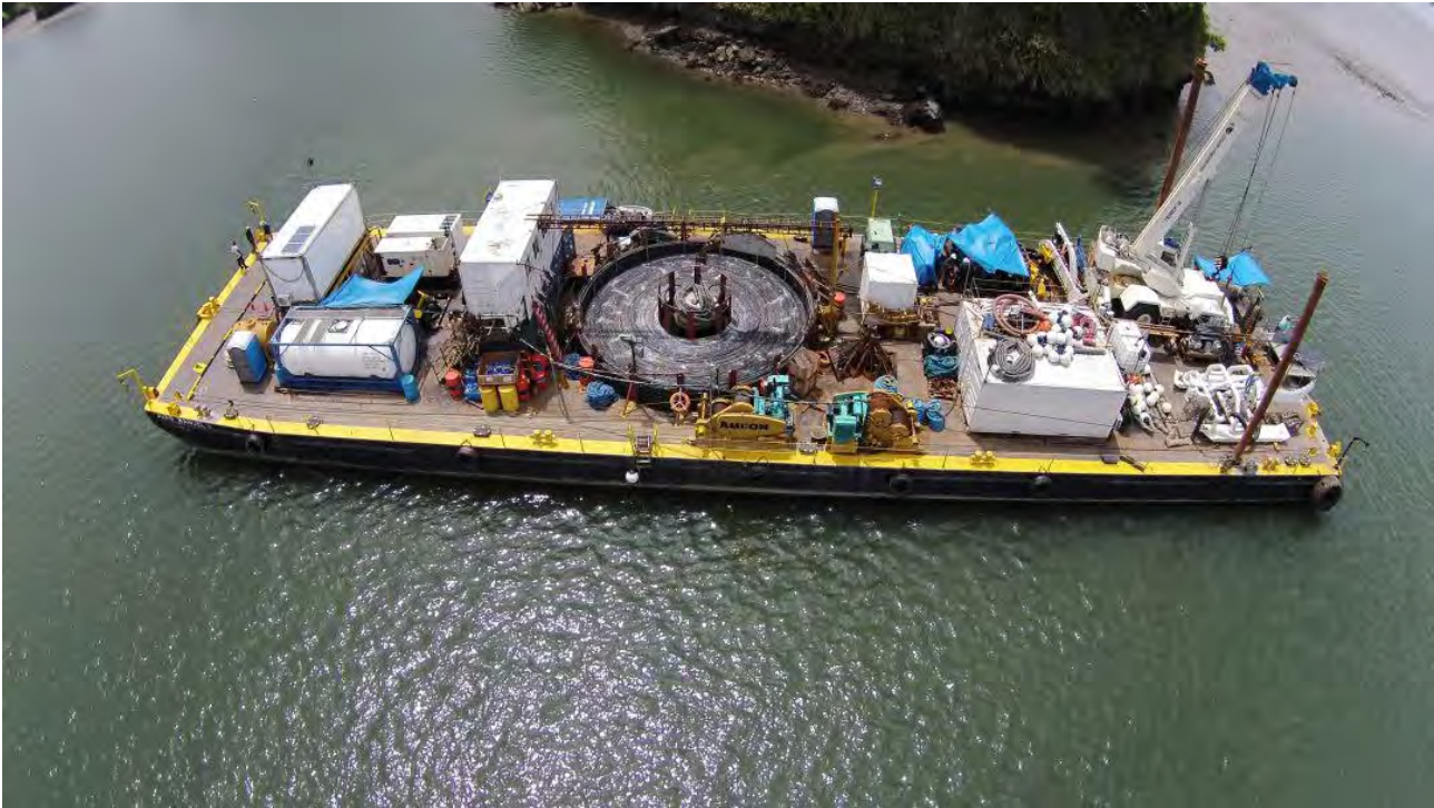
Figure 2-51. Example of cable lay barge (Source: Geomares)
