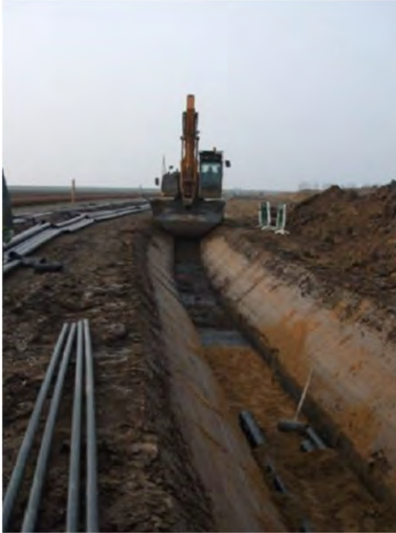
Figure 2-36 – Photo of sub soil excavation in a trench with side slopes (Source: Prysmian)
