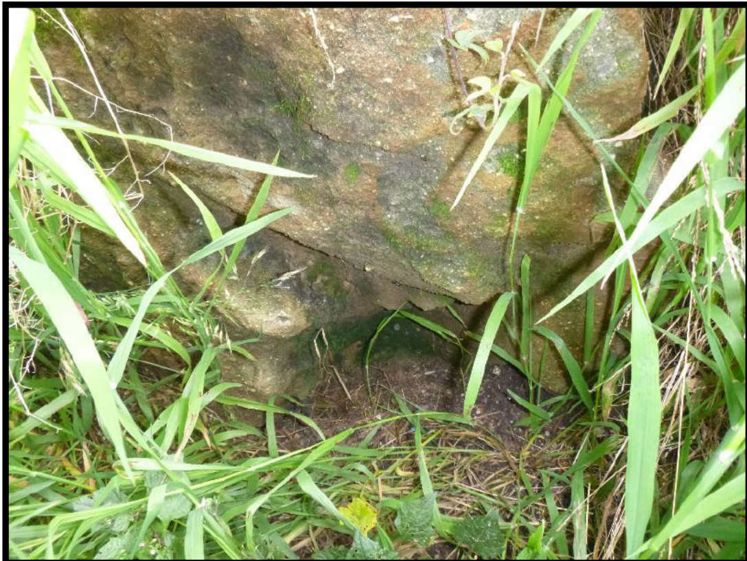
Photograph 16 – Photograph captured 13 October 2021. View of rock outcrop along the southern side of the subject land (i.e. long 1 Campbell Grove boundary). No evidence of loose / displaced soil at the toe of the rock outcrop.
